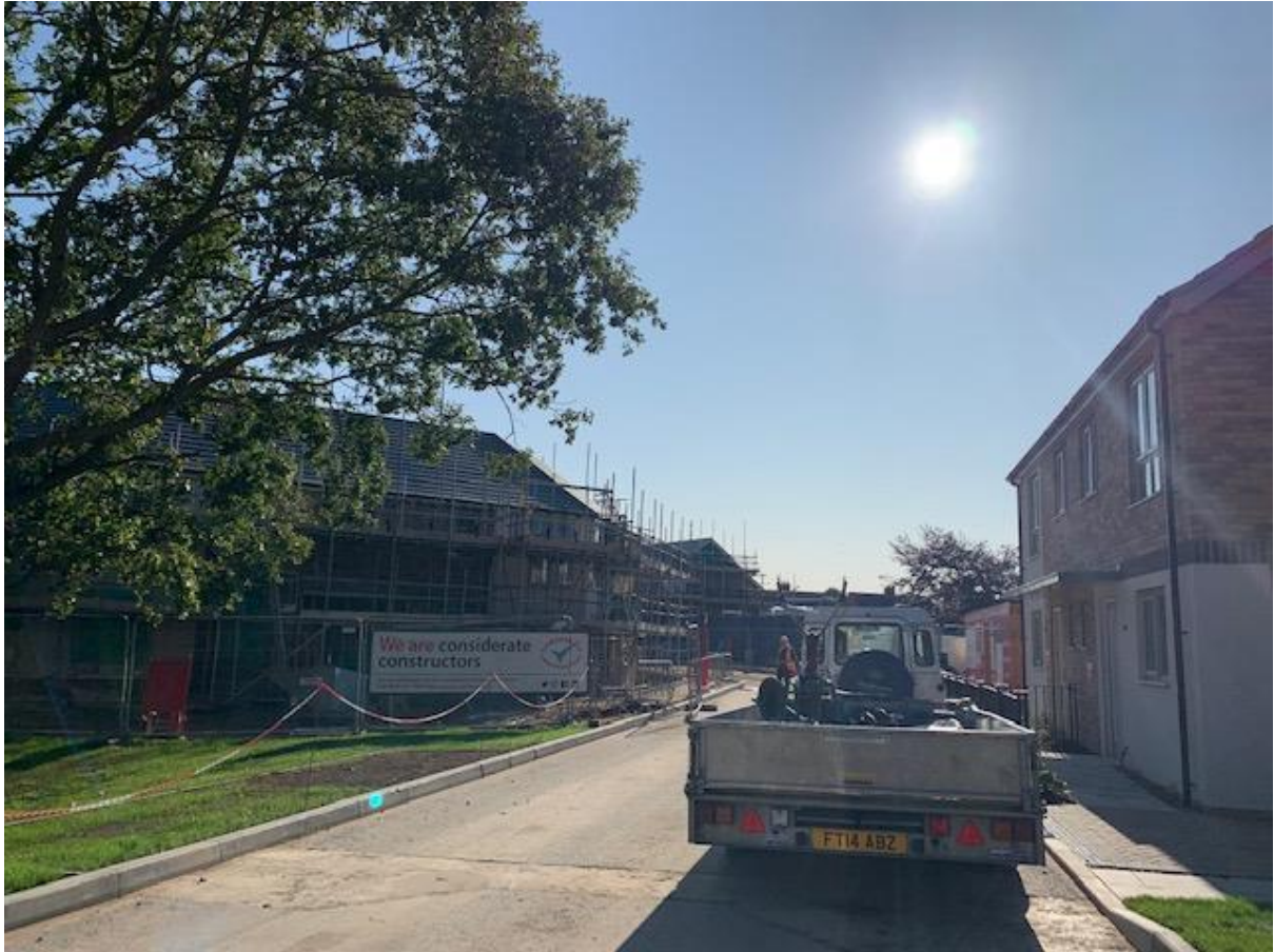
Photo to show construction work currently being undertaken at Phase 3
